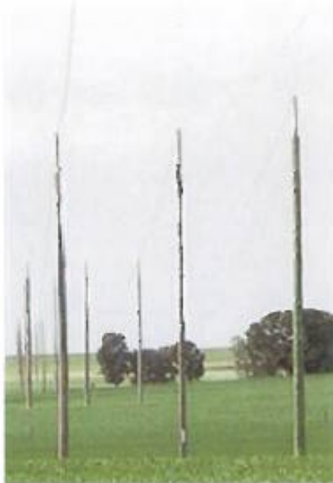
Figure 2.3: Cricket Wicket Wood Pole Power Line
